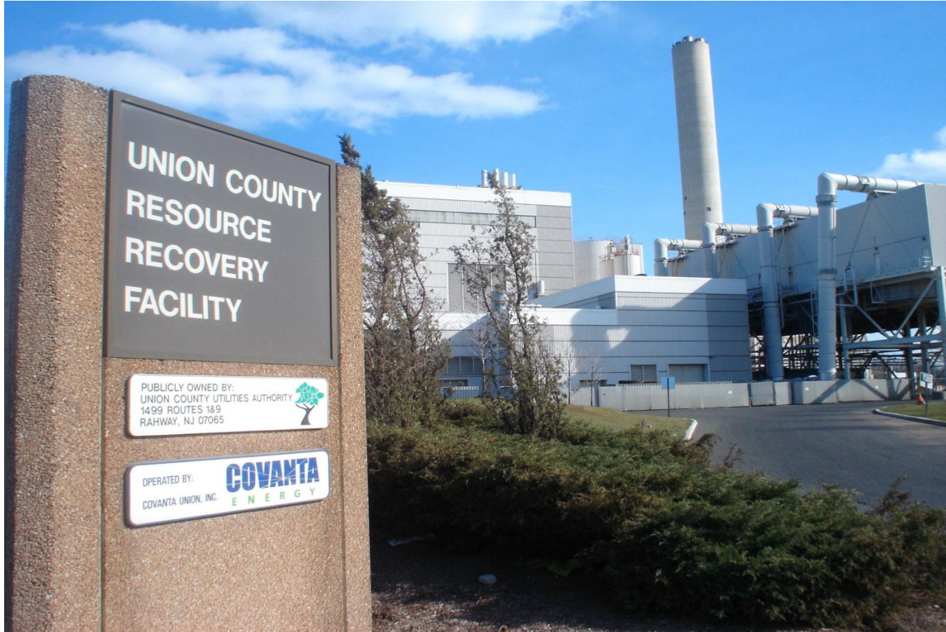
UNION COUNTY RESOURCE RECOVERY FACILITY
