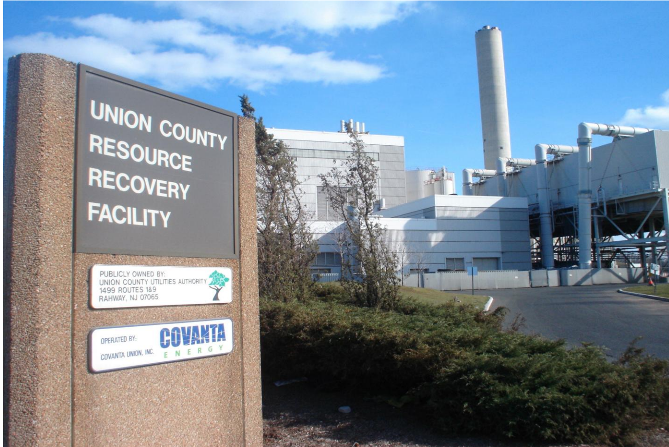
UNION COUNTY RESOURCE RECOVERY FACILITY
